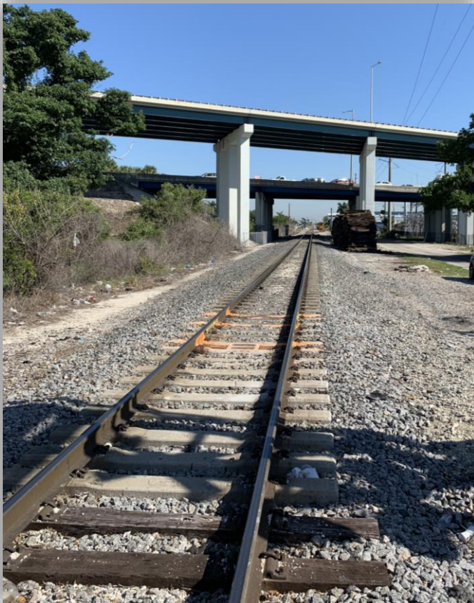
Existing Single Track
